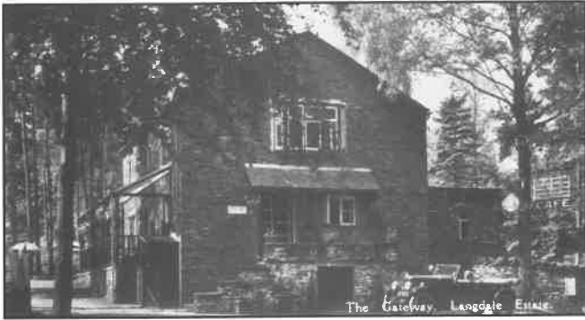
Simple life: cabin dwellers could get a cup of tea and a bath here
