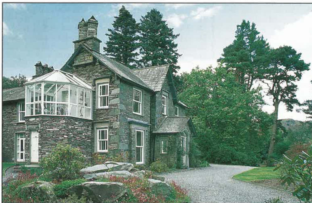
Winter fuel: Elterwater Hall's traditional Cumbrian chimneys are from an age before central heating
