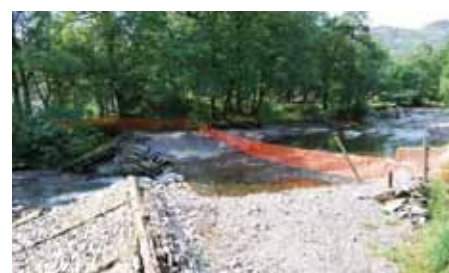
The Weir 2010 - Work starts to repair the damage
