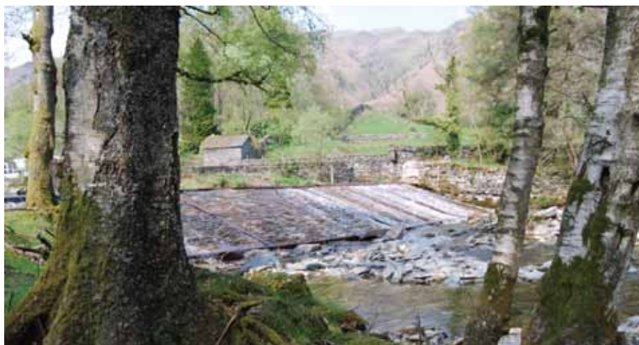
The Great Langdale Beck Weir now restored to its original glory
